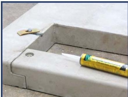
SPLIT PADS FOR REPLACEMENT
