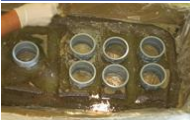
Spread the InstaGrout with a stick
