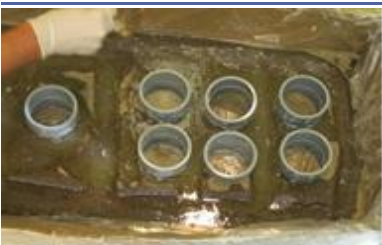
Spread the InstaGrout material with a stir stick
